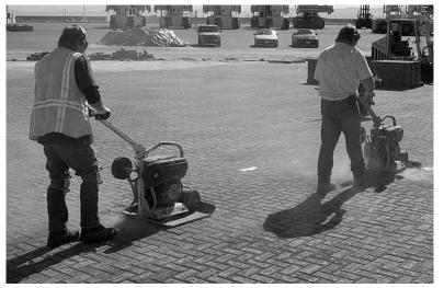
Figure 9. Initial compaction sets the concrete pavers into the bedding sand.
