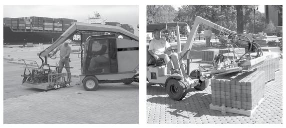
Figure 1. Mechanical installation of interlocking concrete pavements (left) and permeable units (right) is seeing increased use in industrial, port, and commercial paving projects to increase efficiency and safety.
